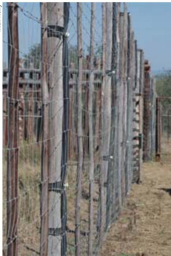
Wholly electrified Bonnox wire mesh fencing on wooden posts with used polyurethane piping and (white) Meps bobbin insulators.
