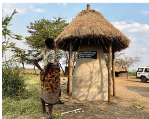
Figure 3. A woman stands in front of an elephant-proof grain store installed by FZS in Tanzania; cement/brick stores like this are used to protect grains from elephants. (© Lucy King/Save the Elephants)
